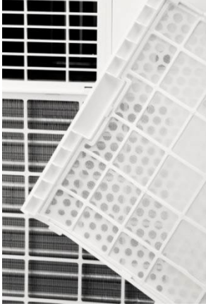
Fig. 7: Switch off the unit and remove the air filter.
